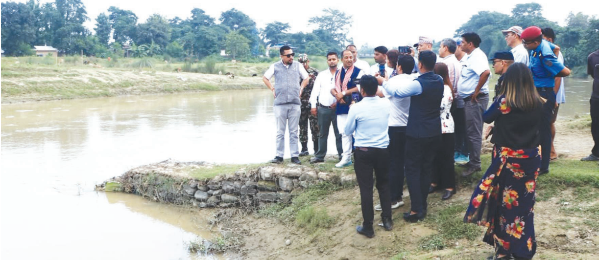
Energy Minister Biraj Bhakta Shrestha inspects the embankment of Sunsari River at Bhokraha Narsingh Rural Municipality-4, Sunsari on Saturday.
