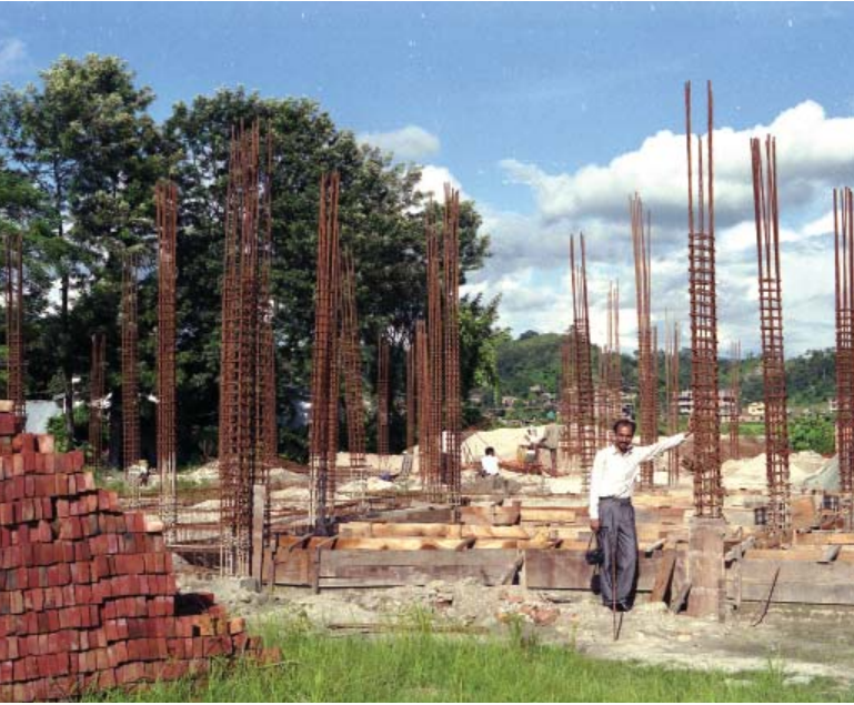
Examples of the strengthening applied to mitigate earthquake damage were tailored to Nepal's specific building styles in 1993.
