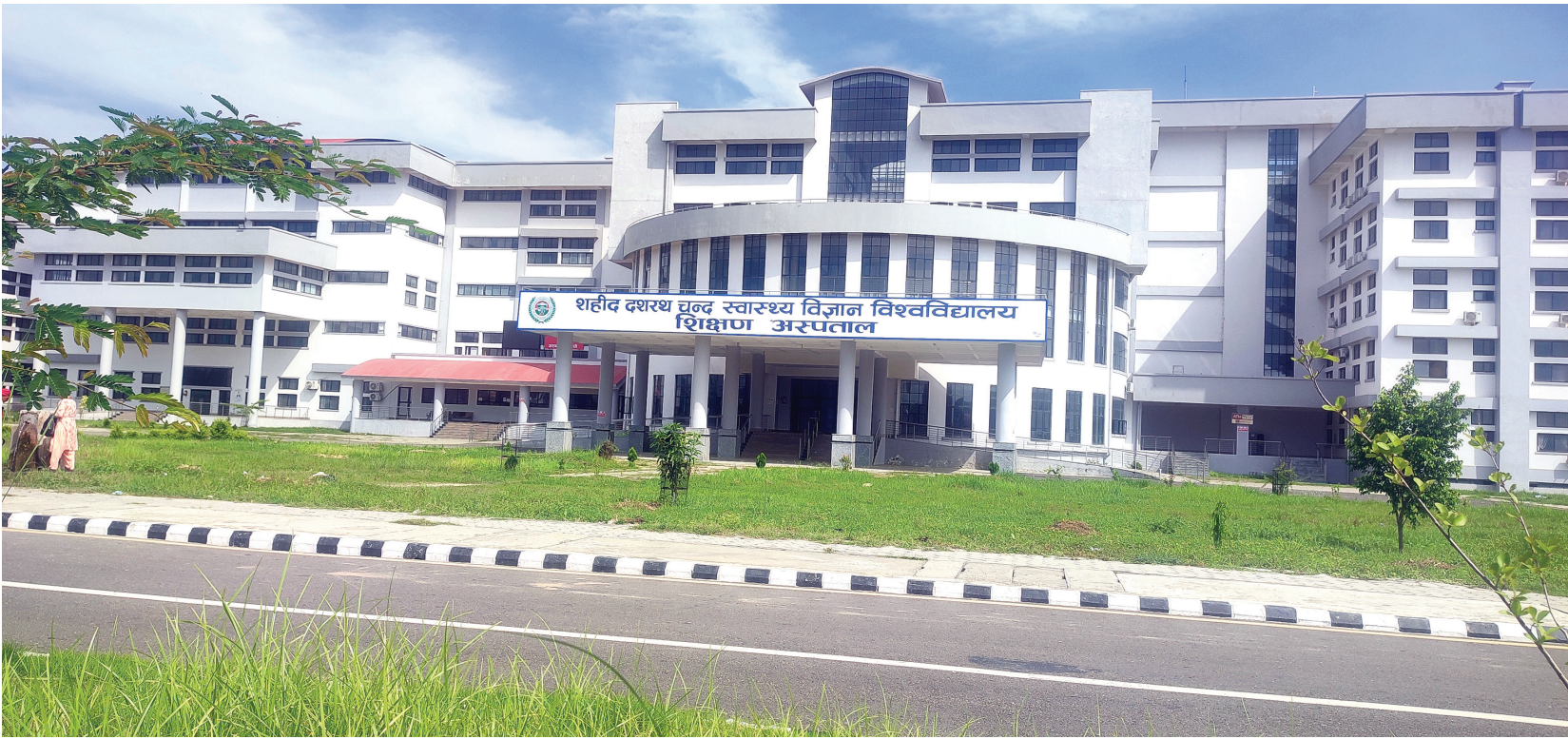
The newly constructed building of Martyr Dasharath Chand University of Health Sciences at Godawari Municipality-5 in Kailali district. PHOTO: RSS
